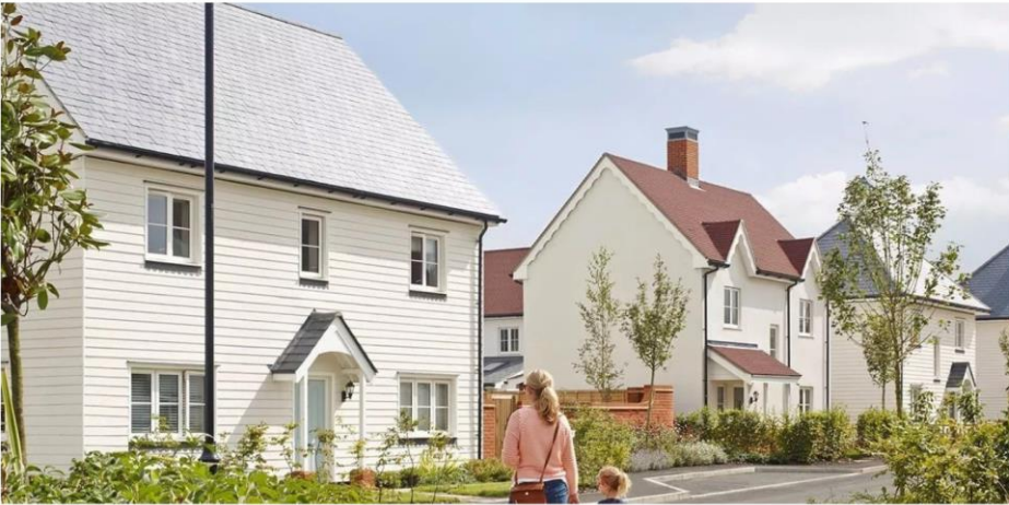
White – render, cladding and painted brick
